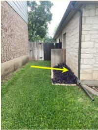
Grade on the south side moves runoff toward the foundation. Other sides had appropriate grading.
